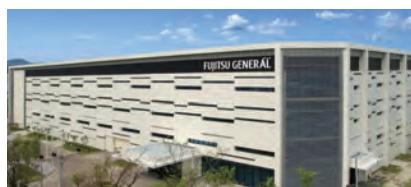
Fujitsu General Air Conditioning R&D (Tajlandia) Co., Ltd. (Tajlandia)
